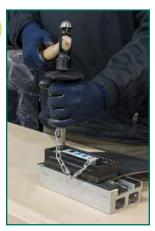
Use a one pound hammer or a pneumatic hammer to set the rivets in the two outside holes first. Continue to set the remaining rivets in any sequence toward the center line. (Tip: be sure all rivets have been set prior to removing the splice from the tool).
